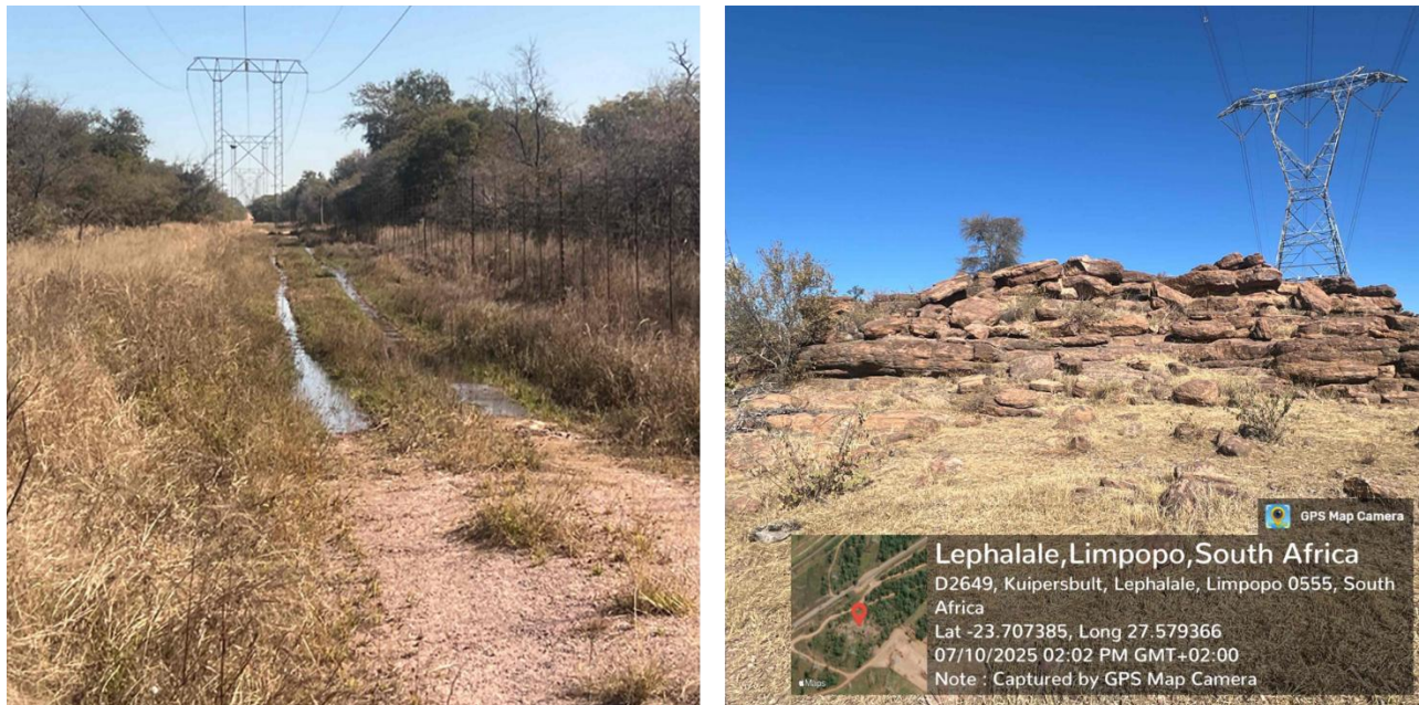
Figure 16: Left – waterlogged area on the Eskom service road where there is an overhead powerline; Right – rocky outcrop/ridge with an overhead powerline.
