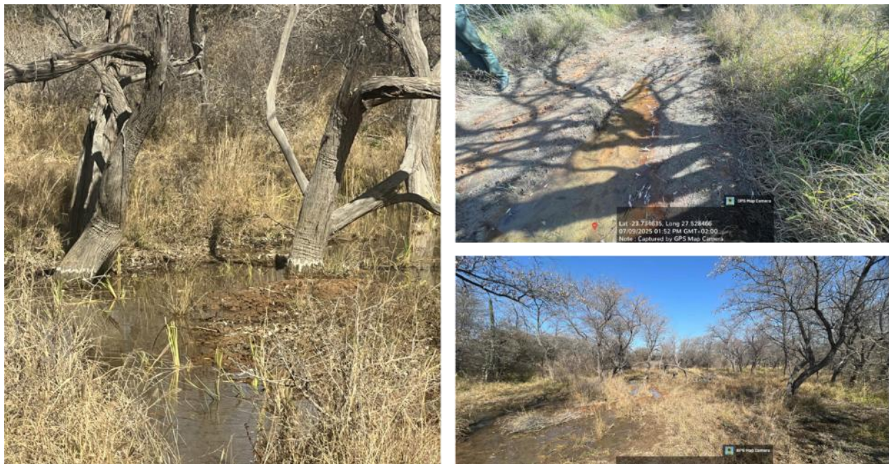
Figure 13: left image – ponding on the site with white residue on tree trunks; Top right – ponding water indicating the presence of iron (brown/orange residue in soil). Bottom right – waterlogged area on the same site.
