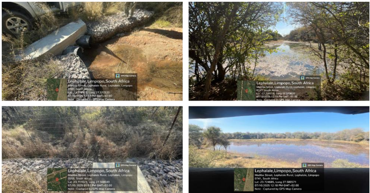
Figure 15: Top and bottom left images – show some of the culvert infrastructure developed throughout the site; Top and bottom right images indicate dams observed on site.
