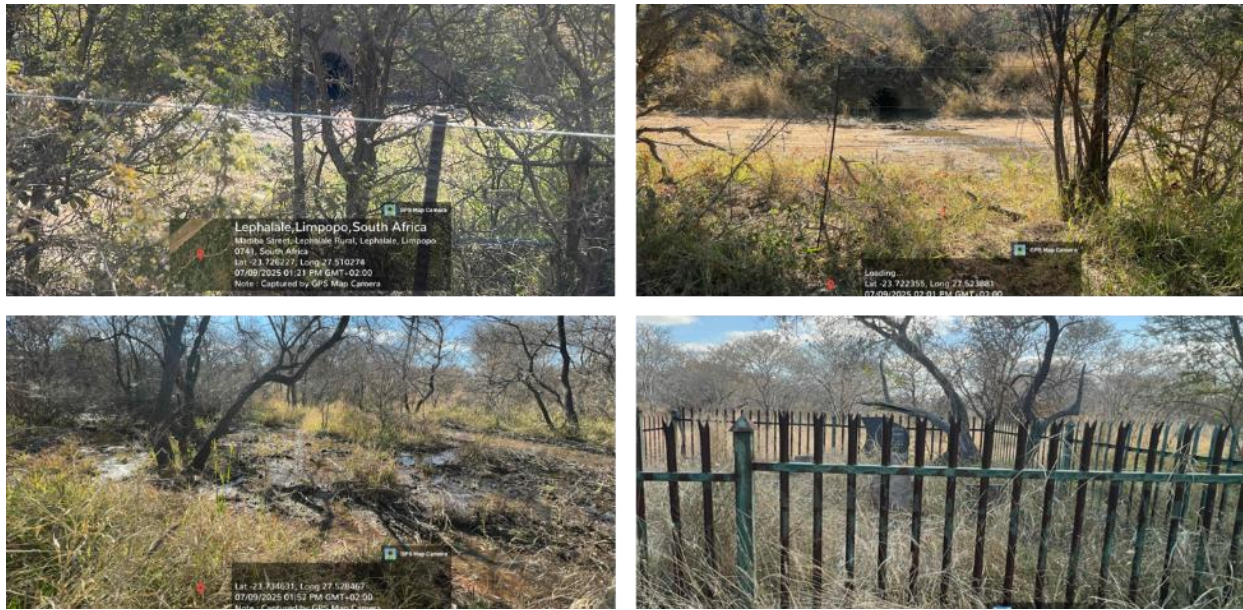
Figure 12: Top left & right – indicates the pipes discharging water into site 1 premises originating from the power station. Bottom left – indicate the marshy features that originate from the water that is coming from the pipelines above. Bottom right – indicates the presence of a grave site.
